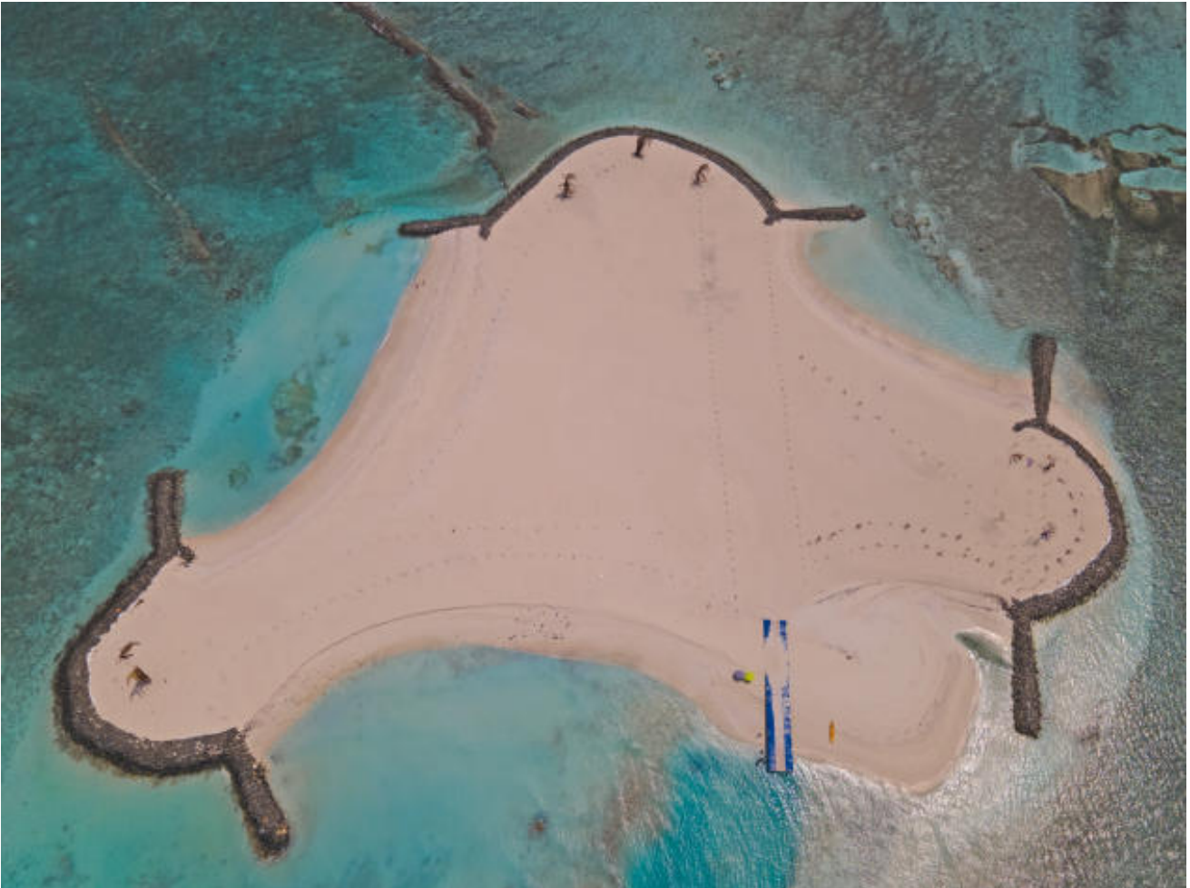
A "picnic" island for tourists and Maldivians was built in the lagoon of Maafushi (Maldives) in February 2022. It is protected from erosion by rocks and some palm trees have been planted. MATHIAS DEPARDON FOR "LE MONDE"
