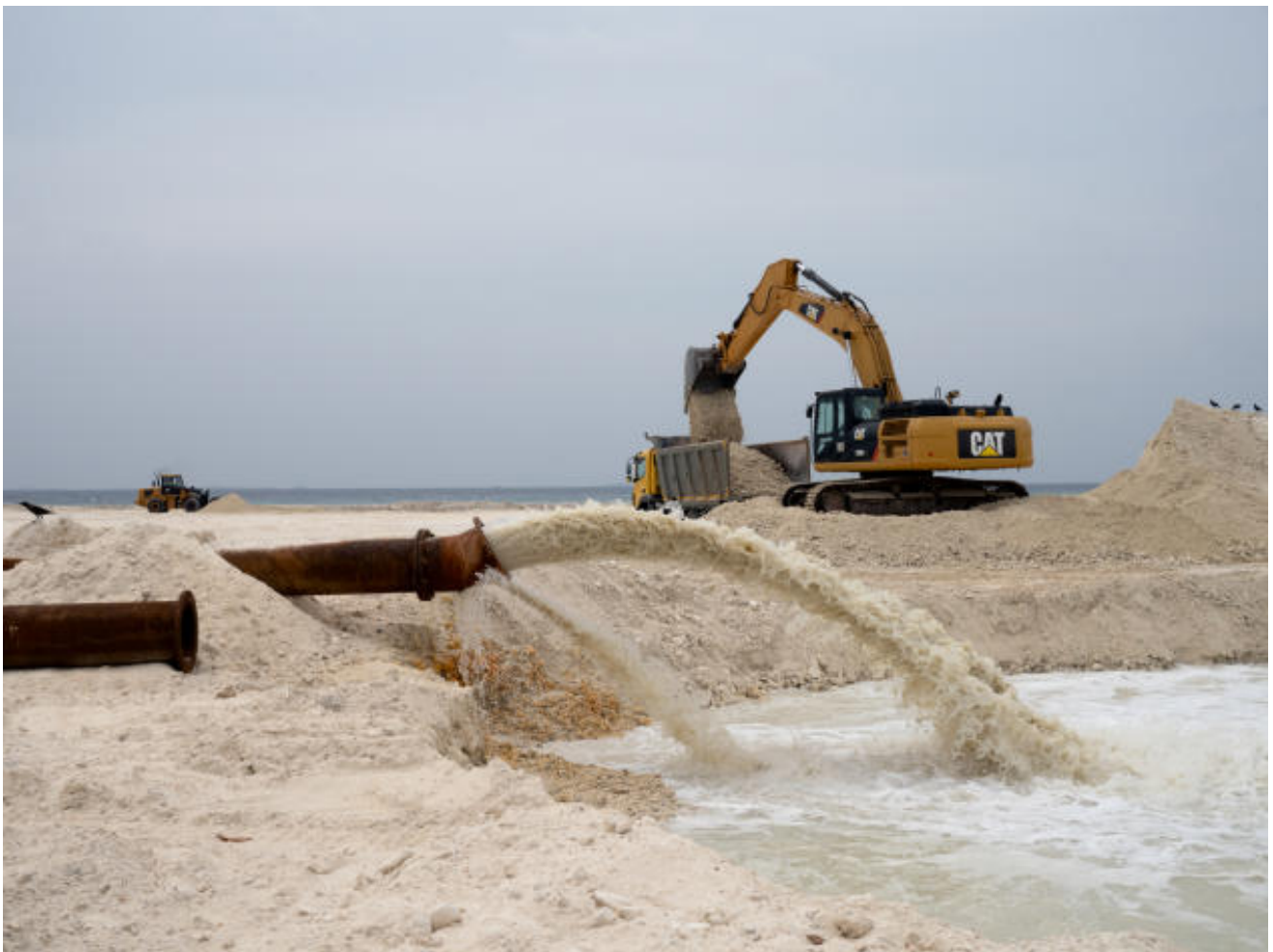
The sand pumped from the bottom of the ocean is continuously spit out on Felivaru Island (Maldives) to fill it in, in February 2022. MATHIAS DEPARDON FOR "LE MONDE"
