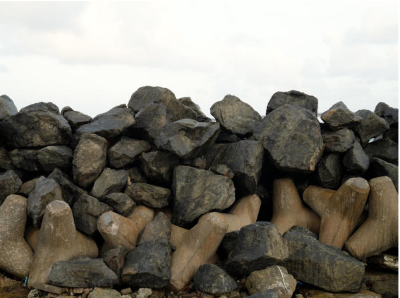
Tetrapods protect the coast of Malé, the capital of the Maldives, on February 6, 2022. MATHIAS DEPARDON FOR "LE MONDE"
